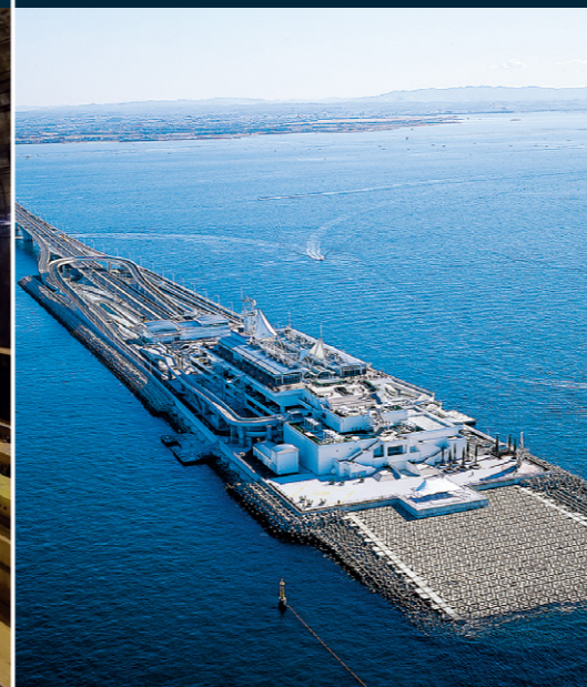
Opened to public in 1997 Tokyo Bay Aqua-Line Umihotaru
