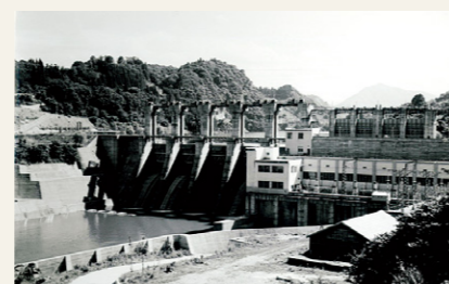
Yanaizu Power Plant
