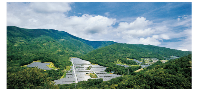
Goyozan Solar Power Plant This plant is located in Goyo-makino, Ofunato City in Iwate Prefecture. The 18 MW power output from a total of 73,440 solar panels is capable of supplying power to the equivalent of approximately 5,800 standard households.
