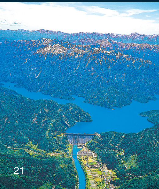
Completed in 1960 Tagokura Dam
