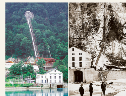
The Takase River power plants sunk into the lake bed for No.2, No.3 and No.4 following a new dam construction a half a century later. The plant No.5 alone was relocated moving the power generation facility which is still in operation today (left).
