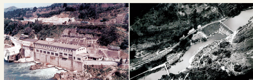
Miyashita Power Plant
