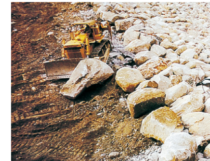
Tilt dozers laid 80,000 pieces of rocks one by one with a diameter of more than a meter to construct the surface of the Takase Dam.
