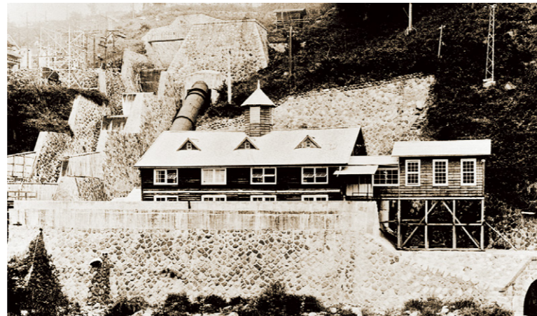
Kiso Fukushima No.2 Hydroelectric Power Plant (Nagano)
