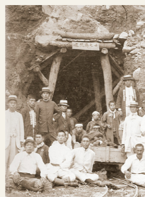
This picture was taken on the Kiso Fukushima power plant construction site. Matabee Maeda sits front and center.
