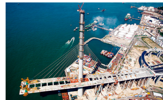
Maeda developed a construction method to build the bridge girders first on the side spans before stretching the girders to the central span due to susceptibility to typhoons and other winds caused by the unbalance between the main towers on the right and left.
