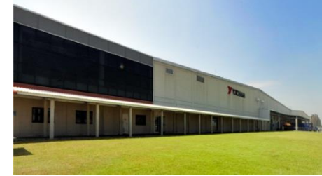
YOKOHAMA TIRE Thailand factory ('09)
