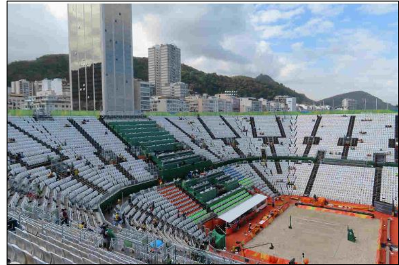
Temporary Overlay Work
