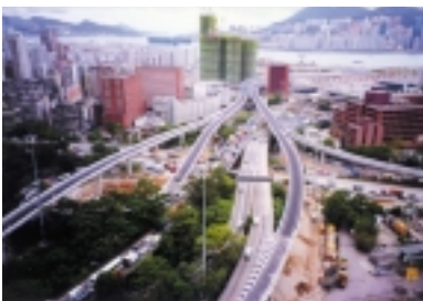
Hung Hom Interchange Bypass
