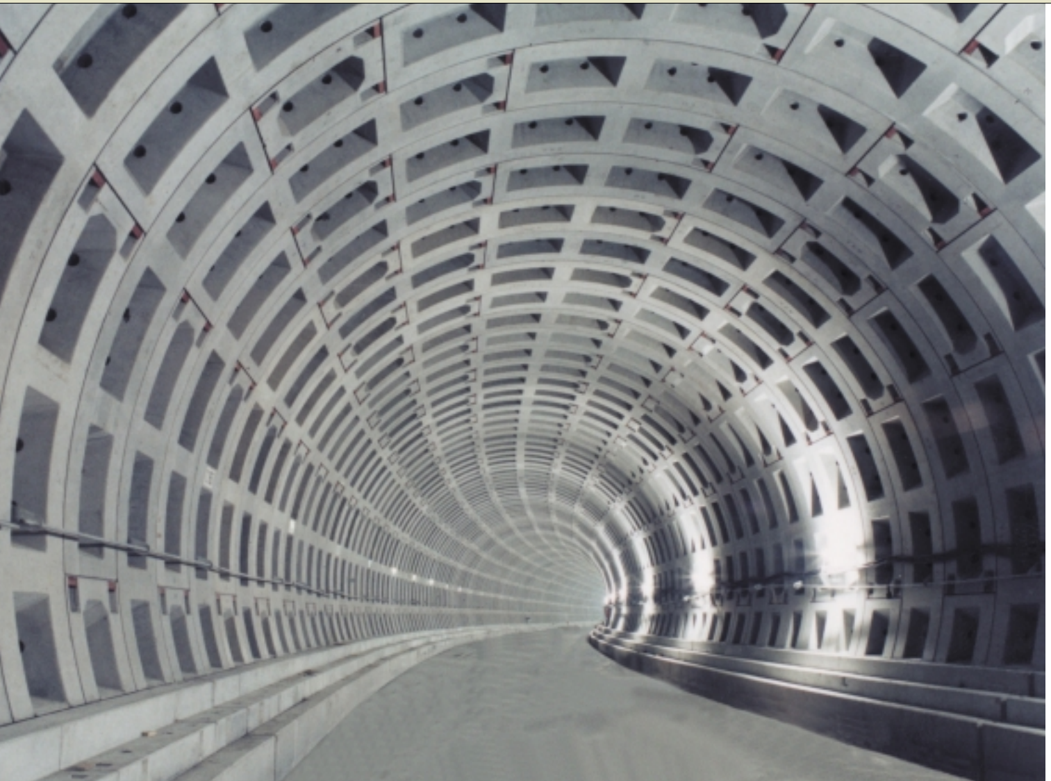
Southern Section of the Kawaguchi Saitama Rapid-Transit Railway—Stage 1 Approximately 1.6 kilometers of mud shielding protect this section of the subway that connects Kawaguchi-Motogo and Minami-Hatogaya.
