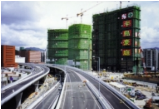
Hung Hom Interchange Bypass
