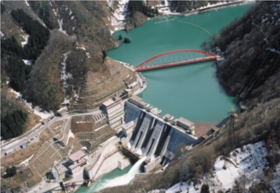
Sixth Stage of Construction of the Unazuki Dam The primary purpose of this 97-meter-high concrete gravity dam is to prevent flooding by controlling the water supply. At the same time, the dam generates power.
