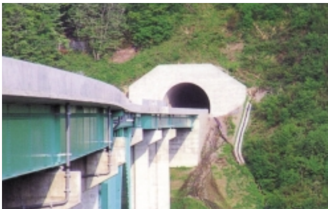
Sekiya Tunnel on the Yamagata Highway This 1,921-meter-long tunnel with a 72m 2 cross-section is outside Asahi Village in Higashi-Tagawa, Yamagata Prefecture.
