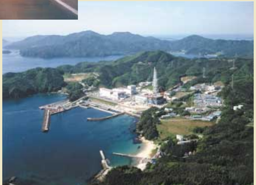
Construction of a condenser used for cooling as part of the construction of the number three reactor at the Onnagawa nuclear power plant
