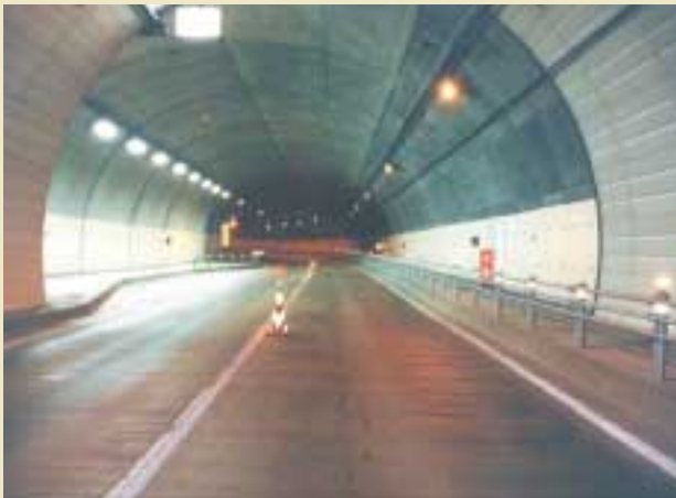
Construction of the Furubira-cho Toyohama tunnel on National Route 229
