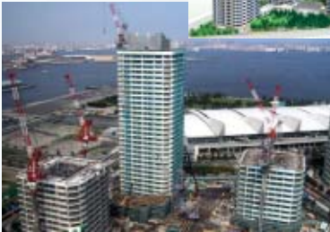
Construction site, April 2002
