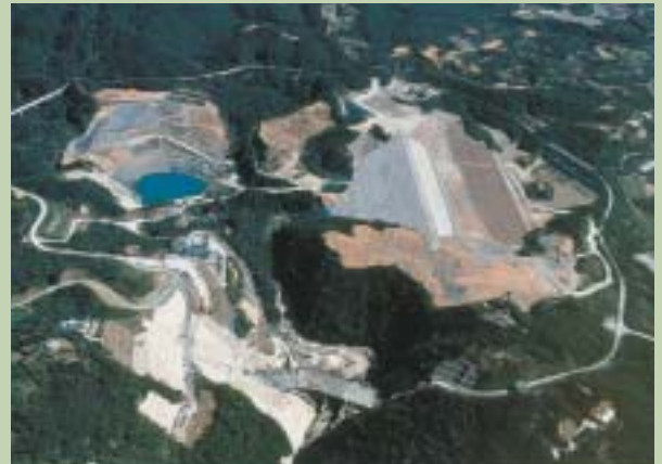
Main Body of the Taiho Saddle Dam
