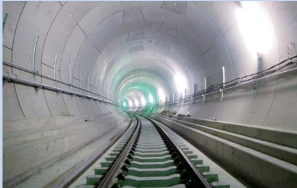
Tokyo Metro Fukutoshin Line: Construction of Subway in Minami-Ikebukuro B-Line Area
