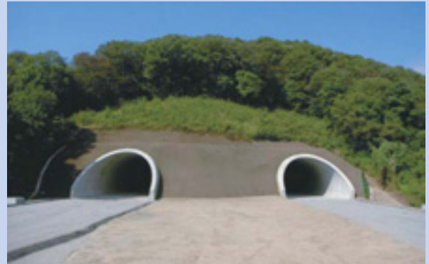
Kita-Kanto Expressway: Construction of Yomogida Tunnel East Section
