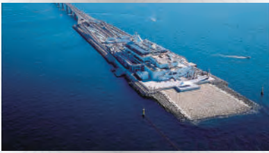
Trans-Tokyo Bay Highway Chiba
