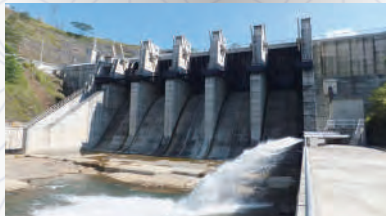
Upper Kotmale Hydropower Project Sri Lanka
