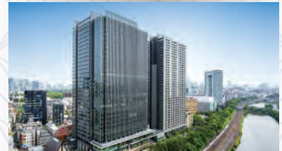
Iidabashi Station West Exit Type I Urban Development Project Tokyo
