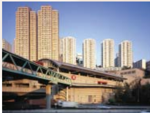
Lai King Station
