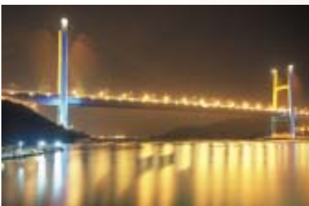
Kap Shui Mun Bridge
