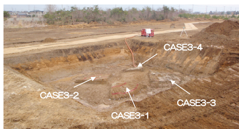
図-15 掘起し改良体全景
