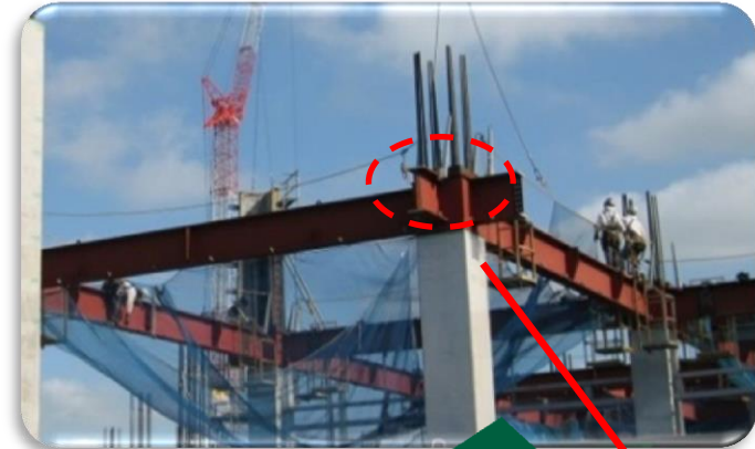
Diaphragm (Cross-beam flange)
