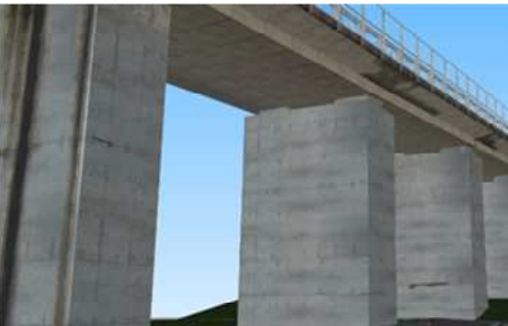
Sanage Green Road
