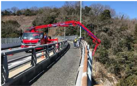
Sanage Green Road
