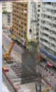
Construction progress as of May 2003
