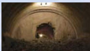
This photo was taken after boring began in January 2003.
