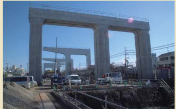
Daini-Keihan (Osaka-Kita Road) Kamimabushi District Support Structures, Etc.
