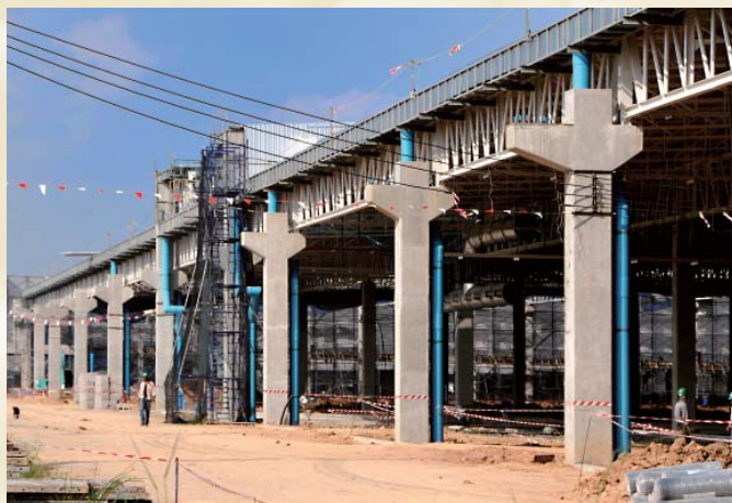
Large rain gutters and spouts to cope with Thailand's powerful rain squalls
