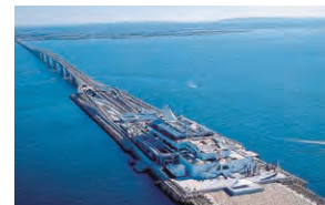
Trans-Tokyo Bay Highway Chiba
