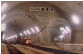
Seikan Tunnel Hokkaido
