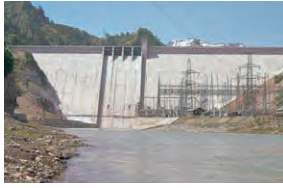
Tagokura Dam Fukushima
